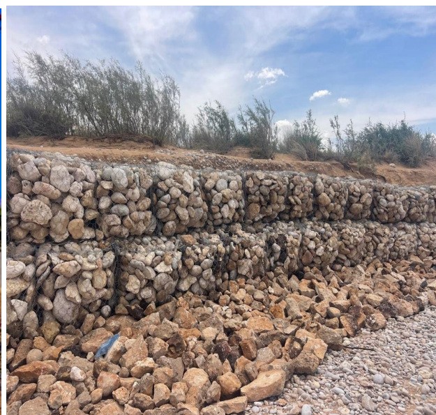
flood protection gabion in EL-dahir, Bari region
